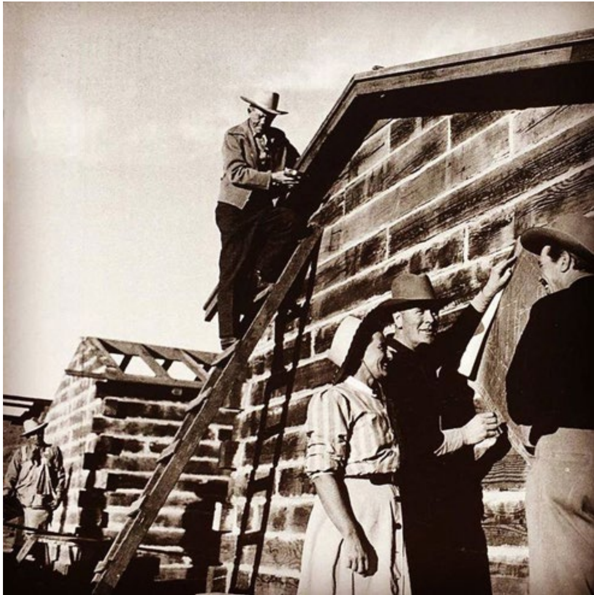
Figure 6. Dick Curtis at far right, building of the Pioneer Townhouse Motel, 1946. Image Courtesy: https://www.pioneertownsun.com/early-photo-gallery/
