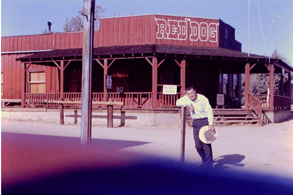
Figure 29. The original Red Dog Saloon, which was lost in a 1966 fire, then reconstructed. View: SW. Image: https://www.pioneertownsun.com/early-photo-gallery/
