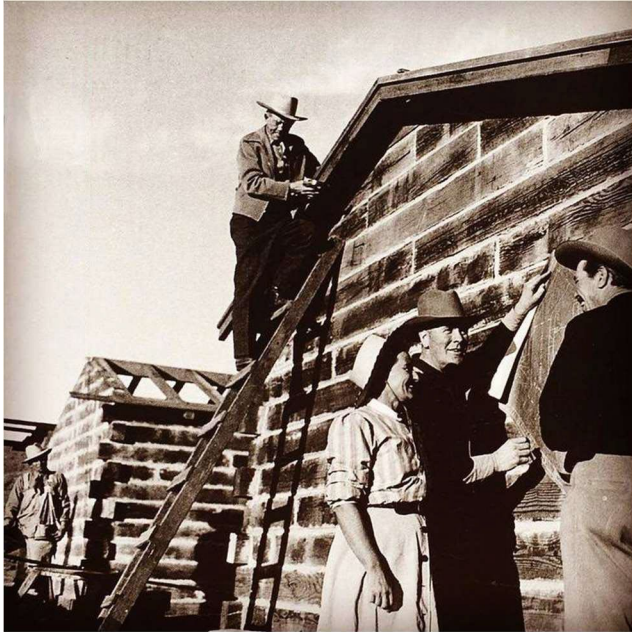
Figure 6. Dick Curtis at far right, building of the Pioneer Townhouse Motel, 1946. Image Courtesy: https://www.pioneertownsun.com/early-photo-gallery/
