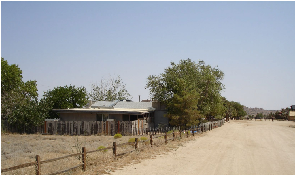
View of the residence on the north side of Mane Street, north of the Project site.
